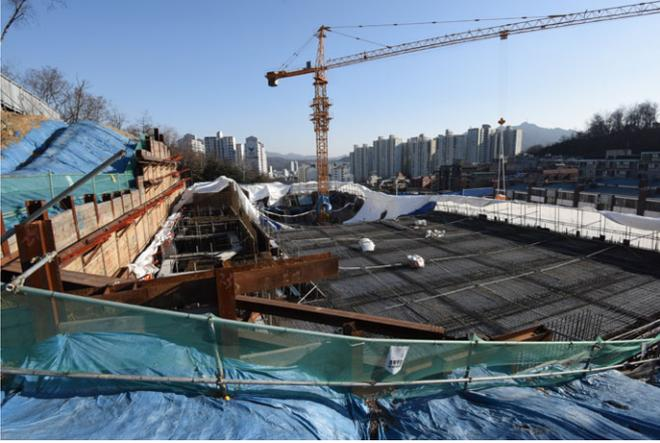
FIG. 1—Top slab of a gymnasium structure. Half of the top slab collapsed while the concrete was being cast, and the other half of the top slab, not cast, did not experience severe damage.
