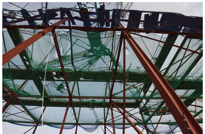
FIG. 9—The collapsed boom, the ruffing jib, and the front and rear struts located on the roof being constructed. The jib angle with the struts remained undamaged.
