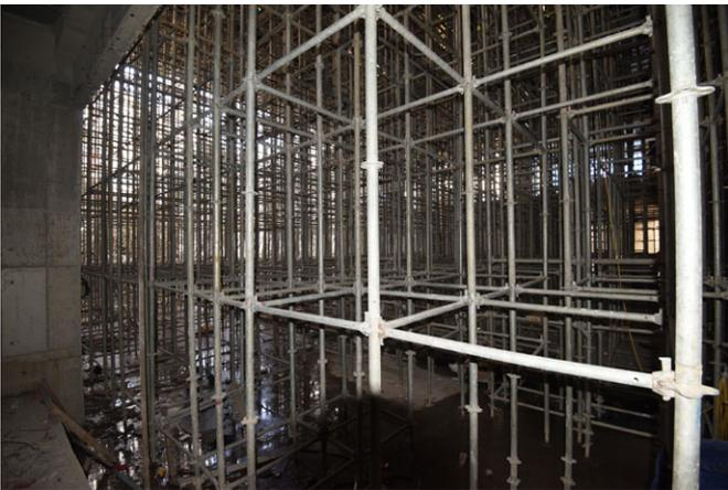
FIG. 3—The remaining prefabricated shore system. It was nearly impossible to check the dimensions of all the remained members of the prefabricated shoring system through the use of a scale because of its complexity.
